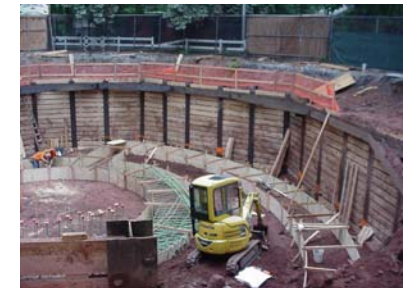
Staten Island Zoo Drilled Soldier Beams and Lagging Shoring System
