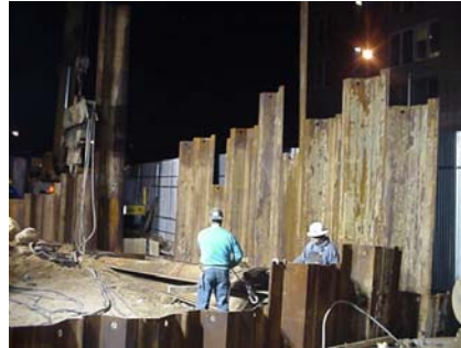
Clara Barton High School UST Tank Removal using steel sheeting
